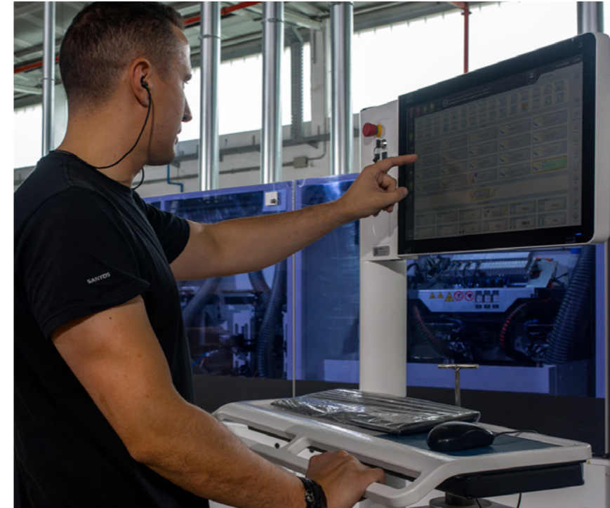
Touch-screens for control and information.
